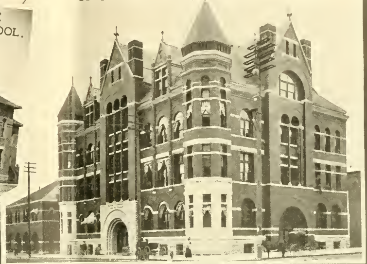
CITY HALL & CENTRAL FIRE STATION.
